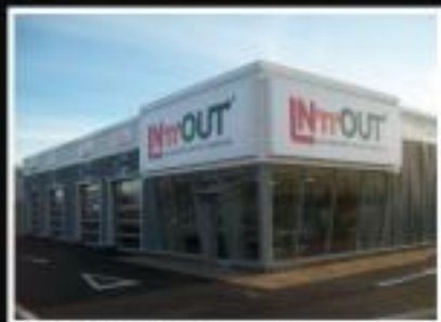
Main I.D. facade signage
