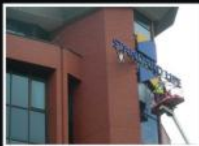
High level main building identification
