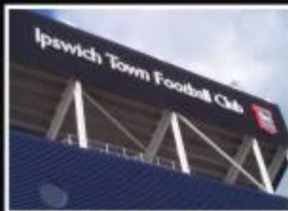
Building identification signage
