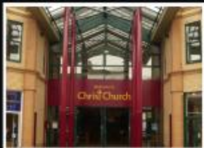
Bespoke facade cladding with individual text
